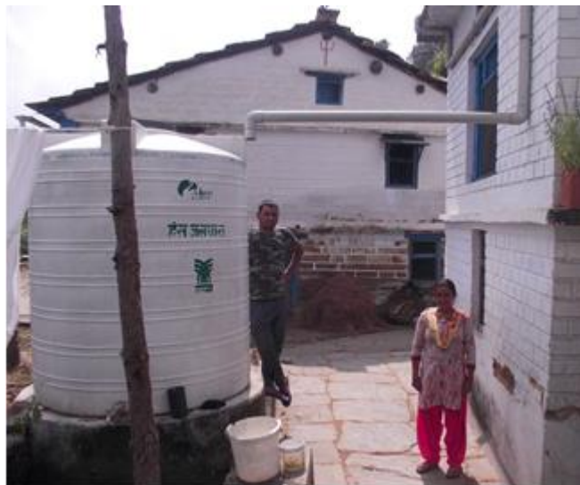
Rainwater Harvesting Tank
